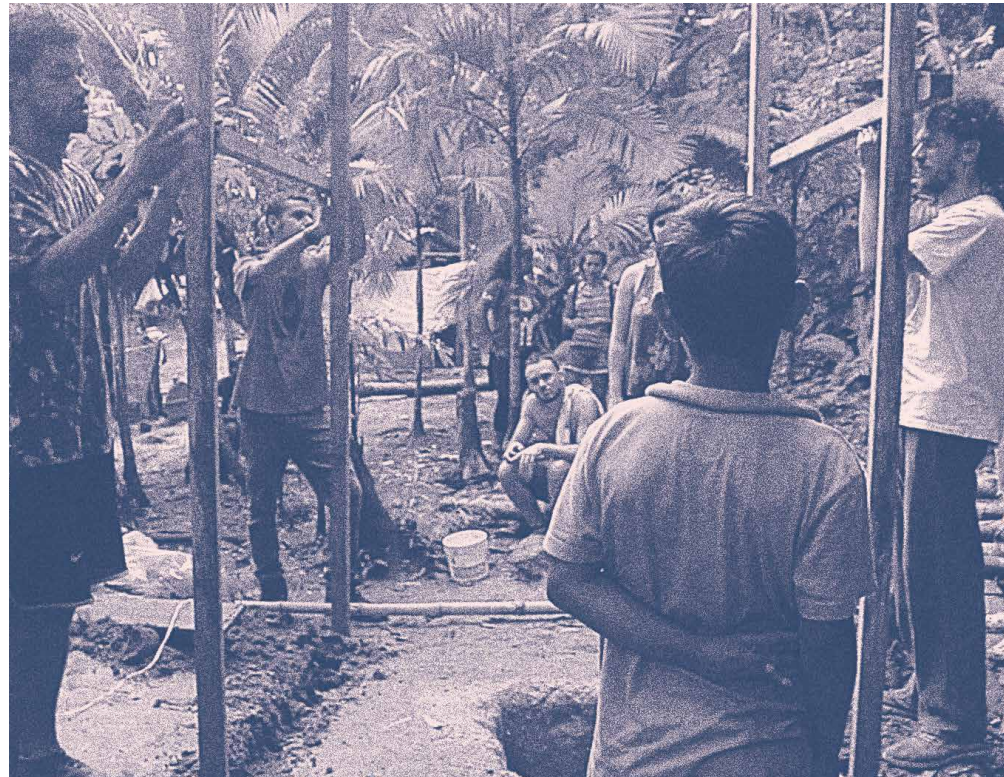
CONSTRUCTION OF THE COMPOSTING TOILET WITH THE GUARANI COMMUNITY, IN SÃO VICENTE
